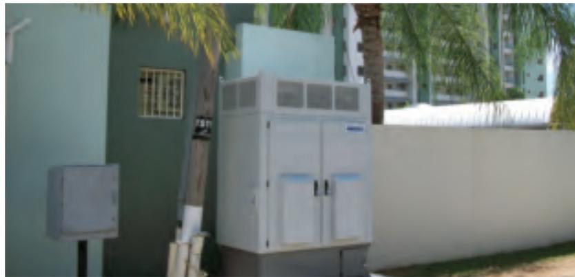
An IdaTech fuel cell sits idle and ready on the island of Trinidad in the Caribbean. But when hurricanes move through the area, it keeps people connected more efficiently and effectively than batteries or diesel-fuel generators.
